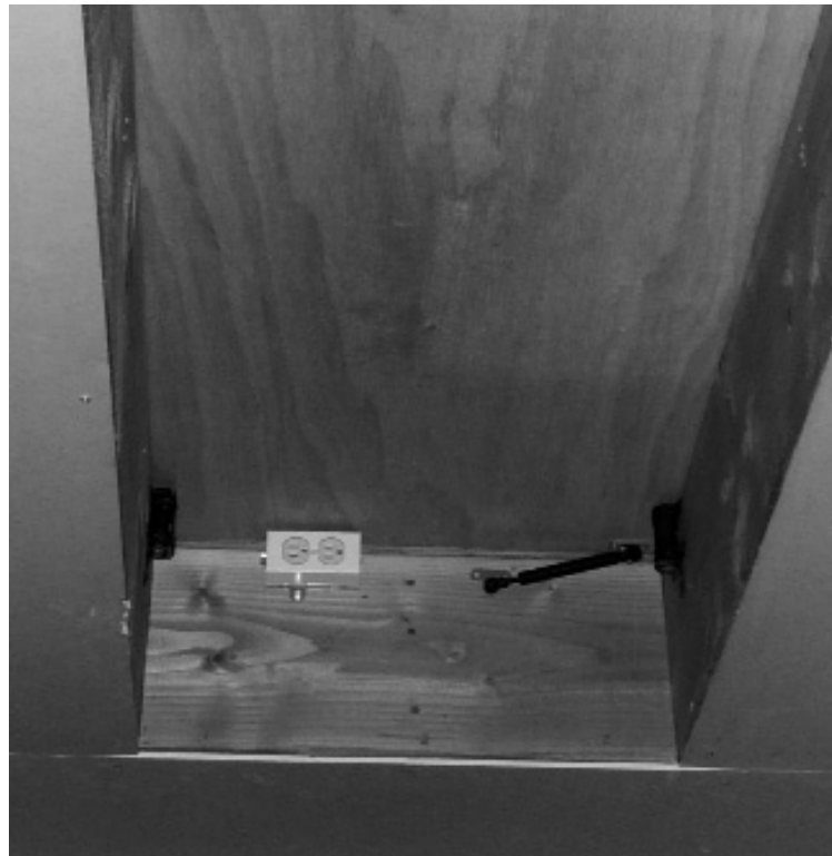
Ceiling Thickness – view with optional floor hatch cover and electrical outlet mounted in rough opening.
